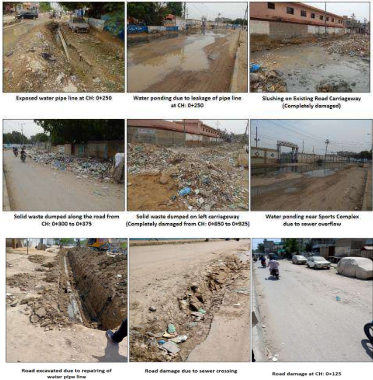
Figure 1-6: Existing Condition of Saudabad Chowrangi to Jinnah Square Road (Nad-e-Ali)
