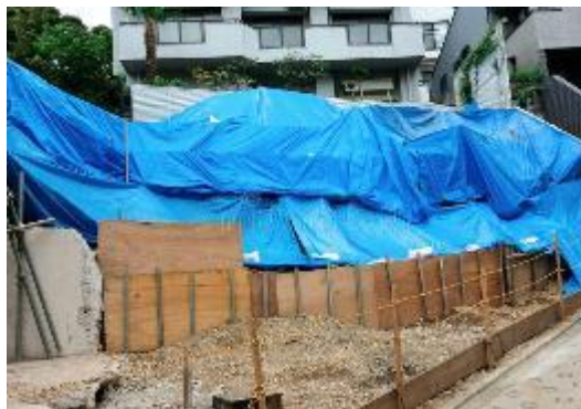
Figure 47: Dust Containment Measures (example)
